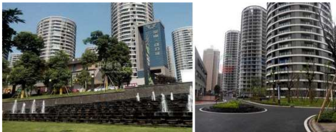
Figure 2.7 Zongshen Motor City Residence in Chongqing (sintered shale hollow brick)
