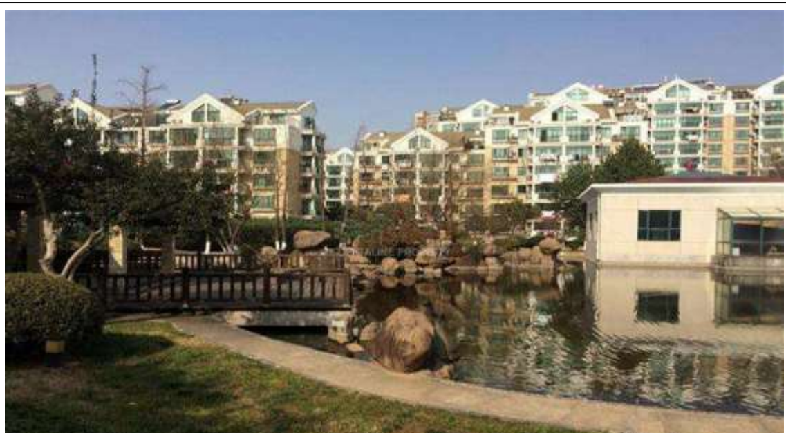
Figure 2.2 Jufuyuan housing estate in Nanjing (shale modular perforated brick)
