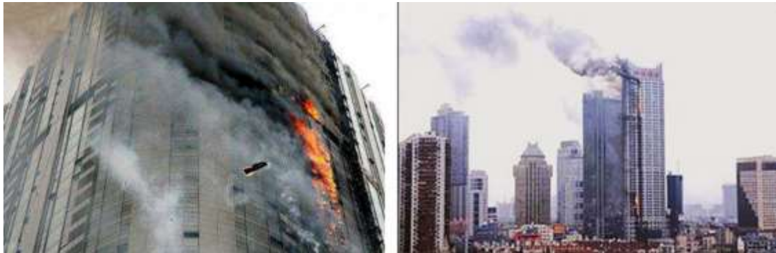
Figure 1.6 Fire disaster at Nanjing Central International Plaza
