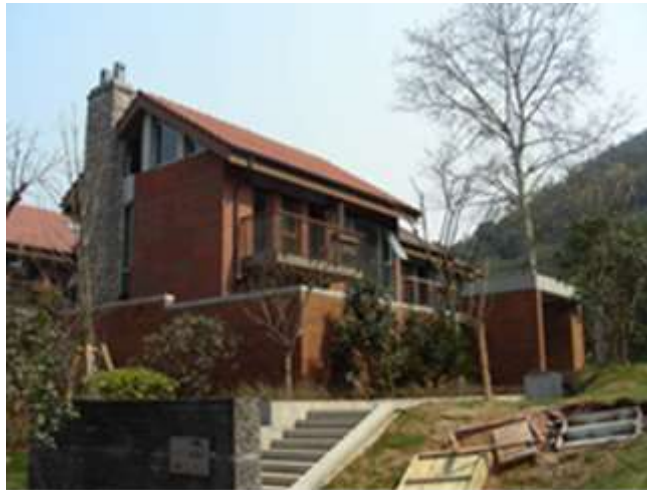
Figure 2.11 Multi-storey terraced house in Kunhe Hejiayuan (sand aerated block)
