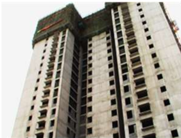
Figure 2.5 Hongkou Hardware Mall in Shanghai (interlocking concrete block)
