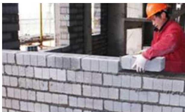
Figure 2.3 Construction of vitrified small ball insulation bricks
