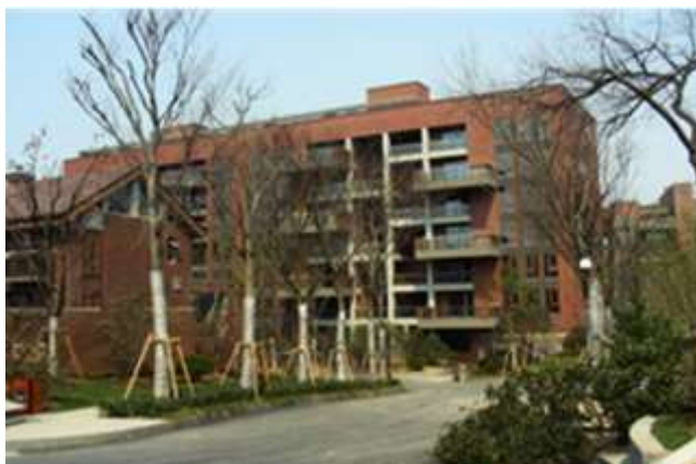
Figure 2.12 Multi-storey apartment in Kunhe Hejiayuan (shale hollow block)
